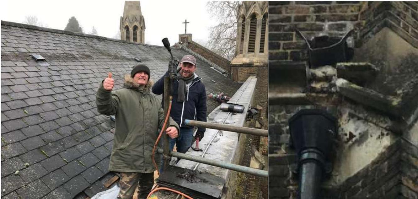
The renovation work is drawing to a conclusion and the additional work to extend the side parapet rain water down pipe and hopper is now in hand. Natural drying out of the interior staining will enable redecoration once the moisture content of the limeplaster has stabilised. Further updates to follow.
